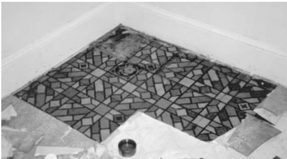
Uncovering the Linoleum.
